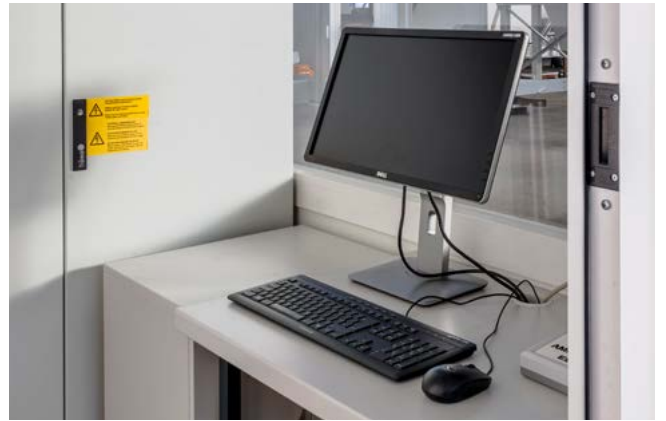
Integrated container with plant control system.
